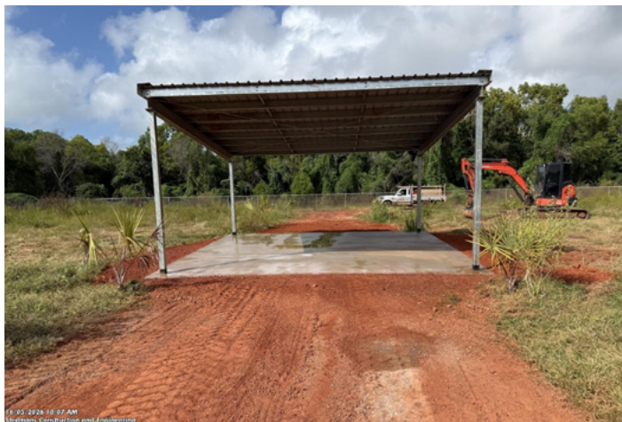
Minjilang Cemetery upgrades include fencing, a shelter, footpath and landscaping.
