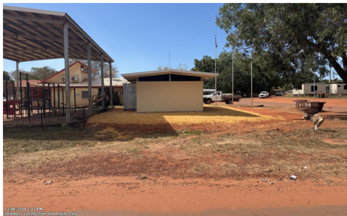
The Maningrida toilet block extension near the Council Office has been completed.
