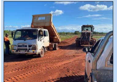
Road repairs have been underway on the Minjilang Airport Road.
