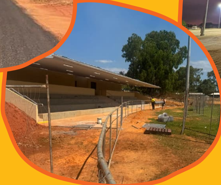
Construction of the new Maningrida Change Rooms.
