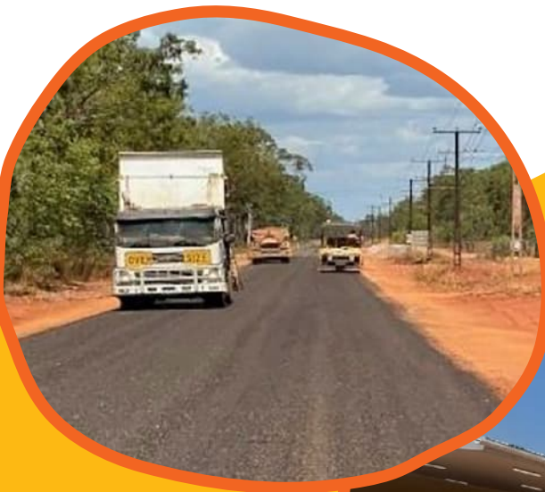
Road upgrades along Malabam Road, Maningrida.
