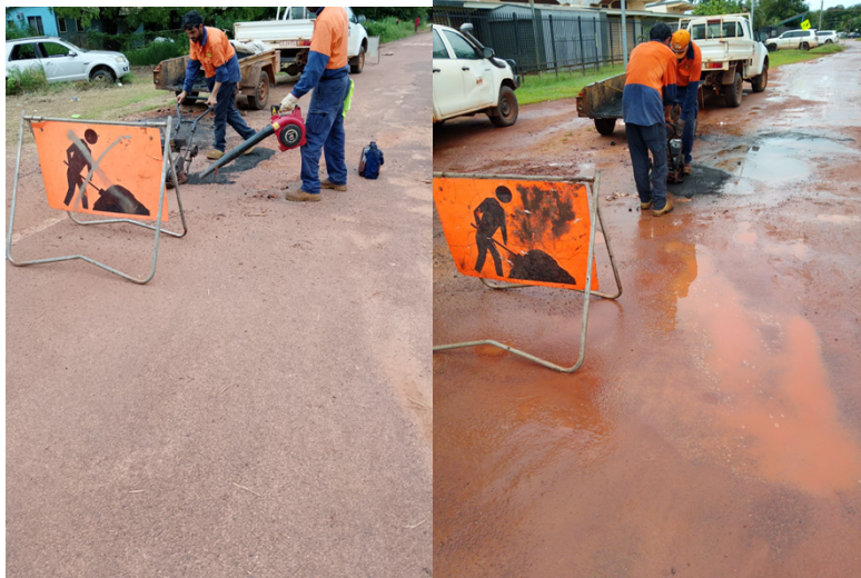
Pothole repairs in Maningrida
