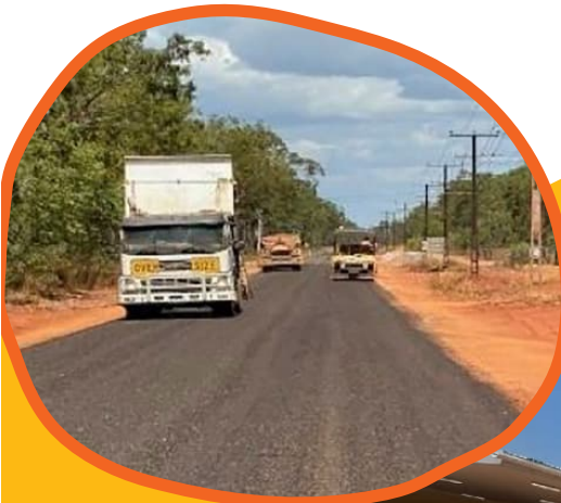
Road upgrades along Malabam Road, Maningrida.
