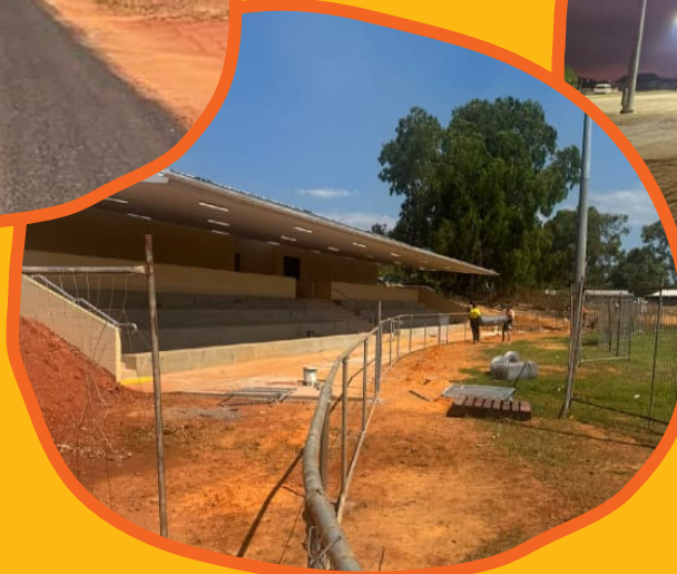
Construction of the new Maningrida Change Rooms.
