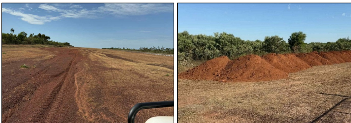
Minjilang Works team repairing wash-out to the airport road.
