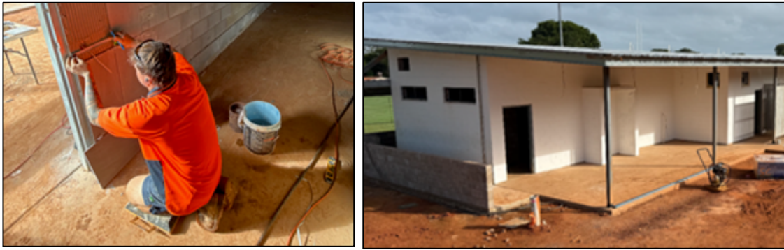
Final touches to the Maningrida Football Oval change rooms.
