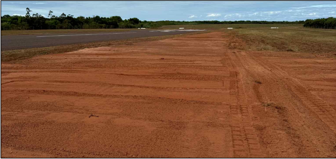
The finish results of repairs conducted to Minjilang the airport road.
