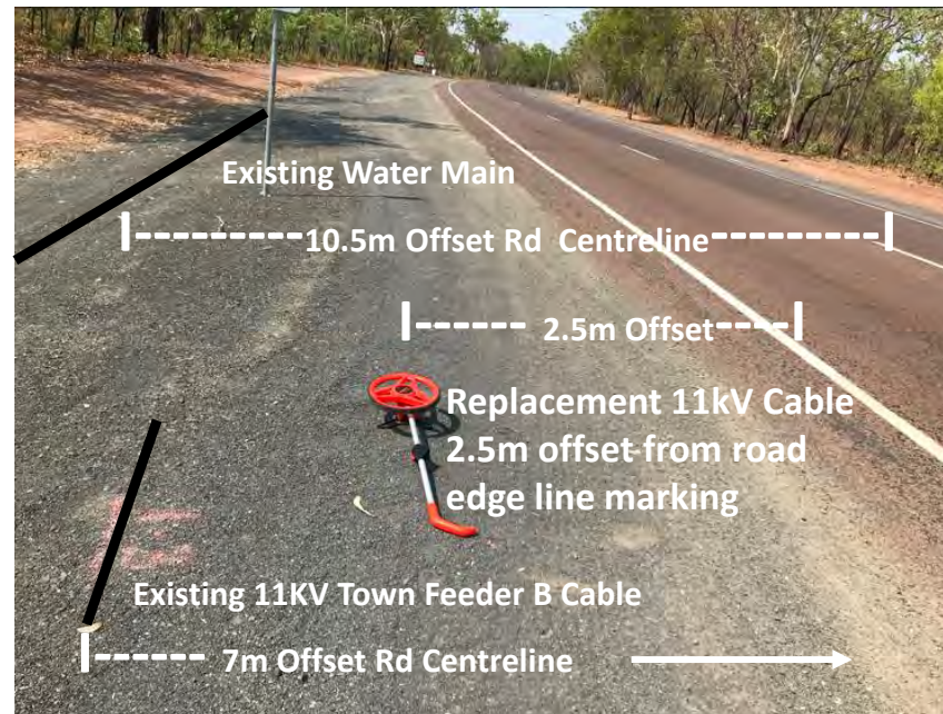
Jabiru Drive northern section Street View looking south. Proposed replacement cable located along the eastern side of Jabiru Drive and within the current service corridor
