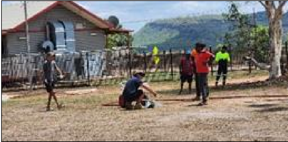
WRAC staff working on resurfacing and irrigation of Gunbalanya Oval.
