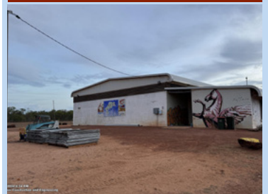
The Waruwi Recreation Hall roofing upgrades are now complete.
