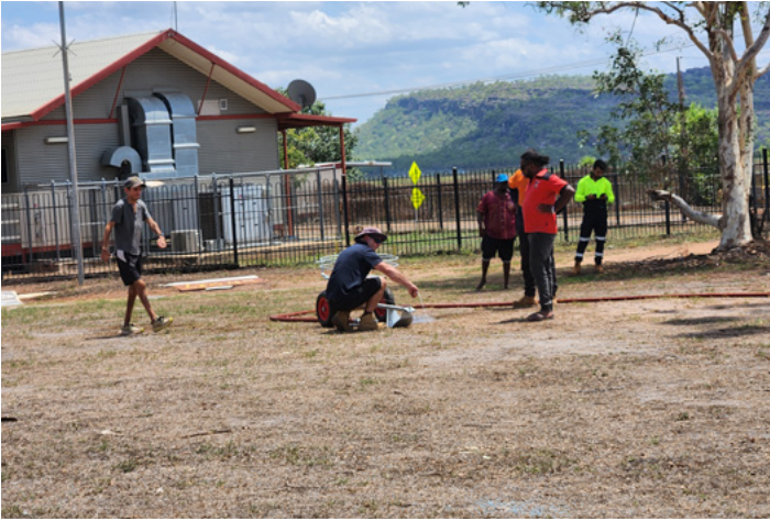
(above) Irrigation upgrades at the Gunbalanya Oval.
