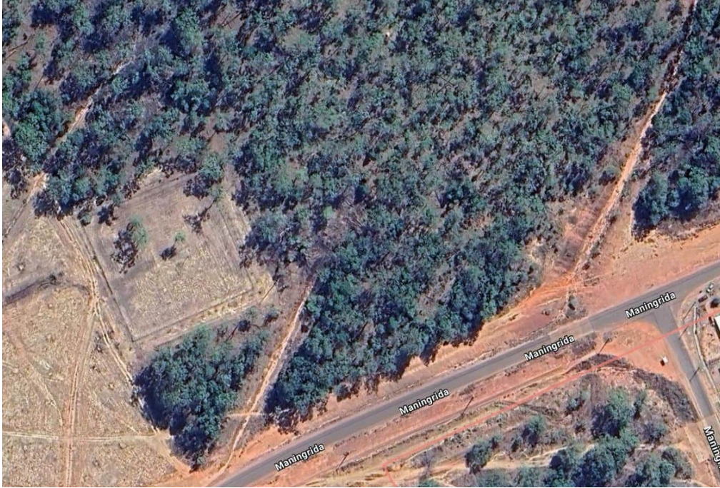
Overhead Current Site
