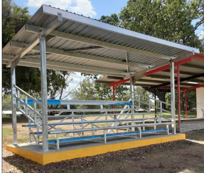
New grandstands at Brockman Oval
