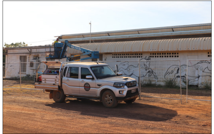
Warruwi Community Hall reroof is underway.
