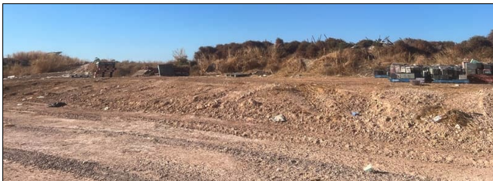
Batteries removed from site – 12.10.24.
