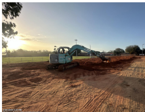
Construction of the Maningrida oval change rooms has commenced.
