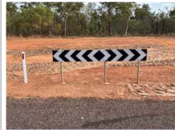
Guide post needs to be turned so reflector faces traffic on road A
