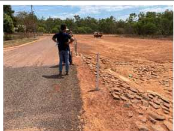
Guide post needs to be turned so reflector faces traffic on road J
