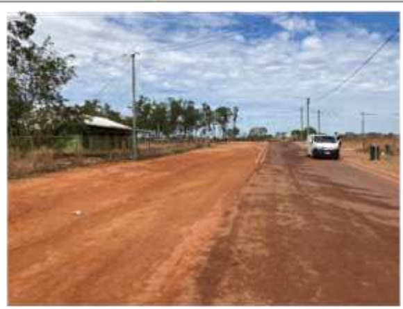
Loose material in TD09
