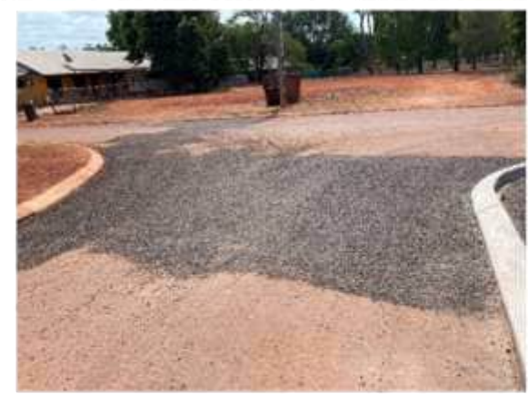
Seal stone to be removed intersection of roads E&F
