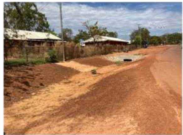
Loose material in TD 04
