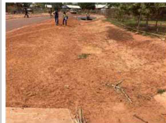
Loose material in TD05
