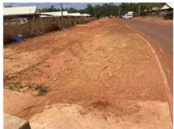
Loose material in TD01
