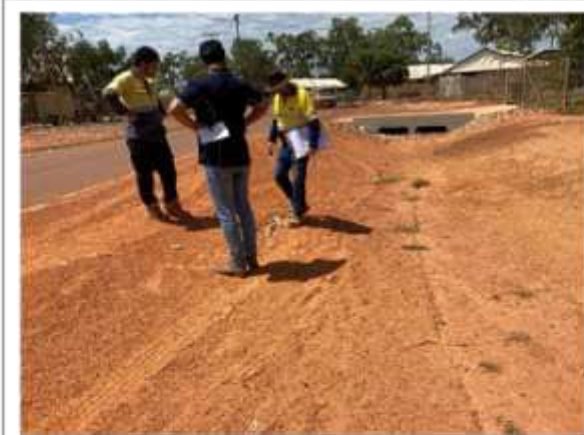
Sub soil exposed in TD05
