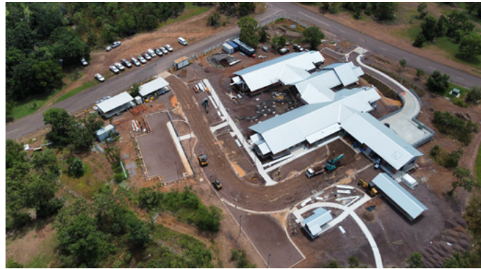
An aerial photo of the new Jabiru Health Centre.
