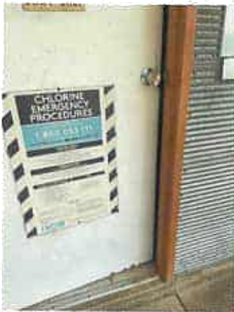
Kiosk door on arrival, partly open
