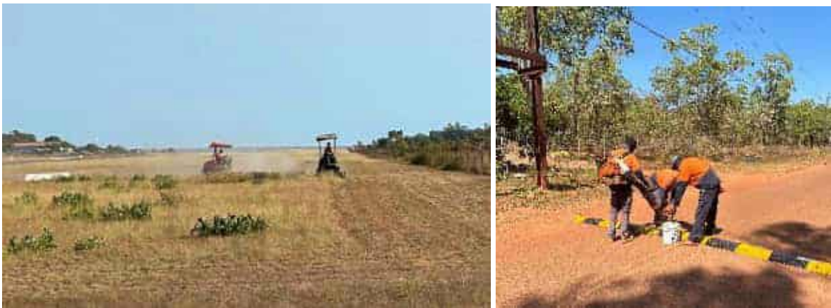
Maningrida aerodrome schedule maintenance and installation of two (2) new speed bumps.
