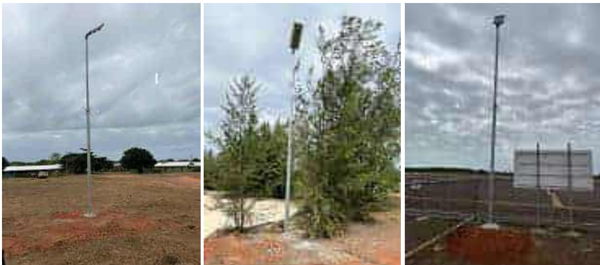
Installation of three (3) new solar lights across Minjilang.
