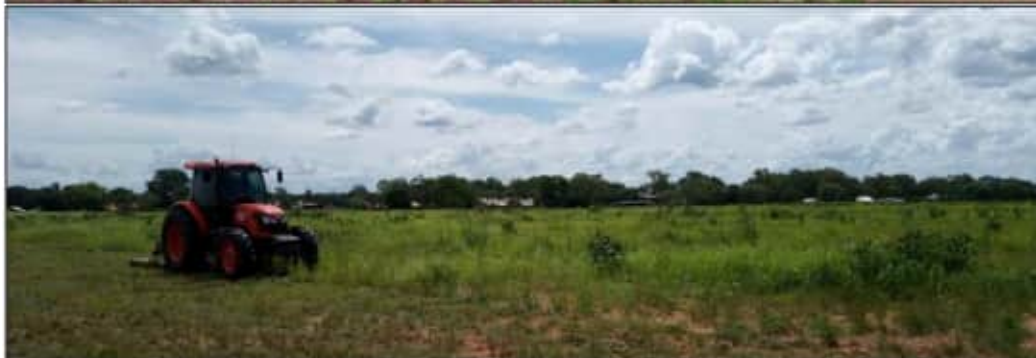
Maningrida works crew have commenced aerodrome ground maintenance.
