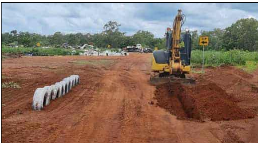
Warruwi landfill site entry.
