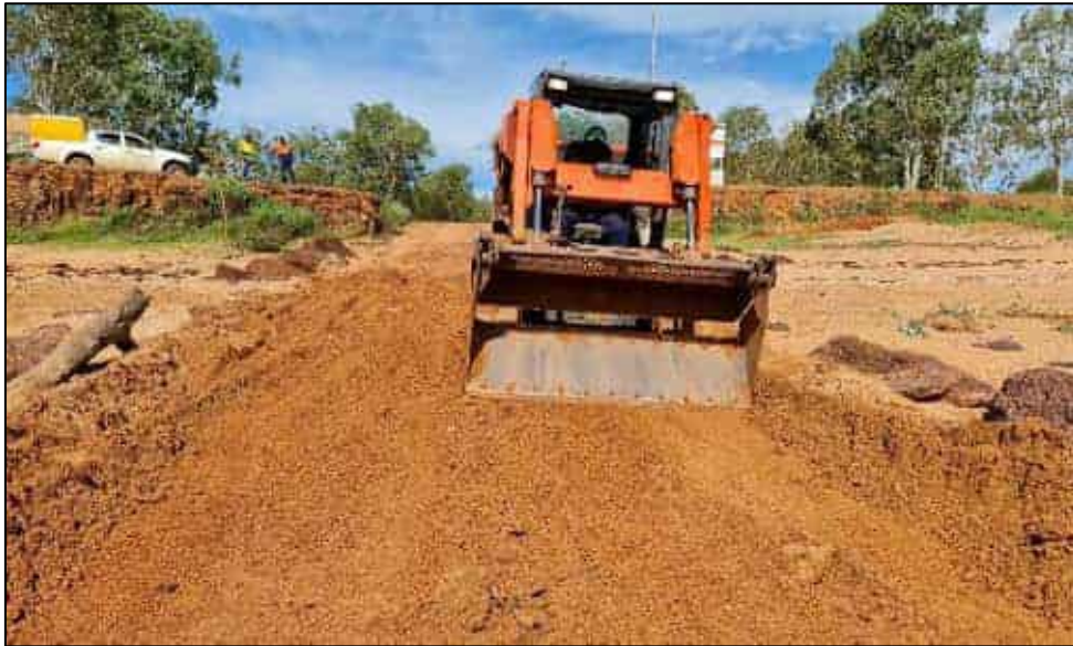
Road works at Fletcher Point.
