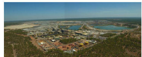
Ranger Project Area aerial
